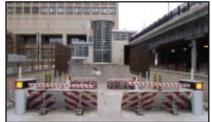
Using decorative concrete bollards and cautionary entrance/exit wedges can easily protect pedestrians on sidewalks and prohibit wrong-way entrance into parking garages. Both of these come from SecureUSA.
